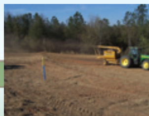
Reseeding the right-of-way
