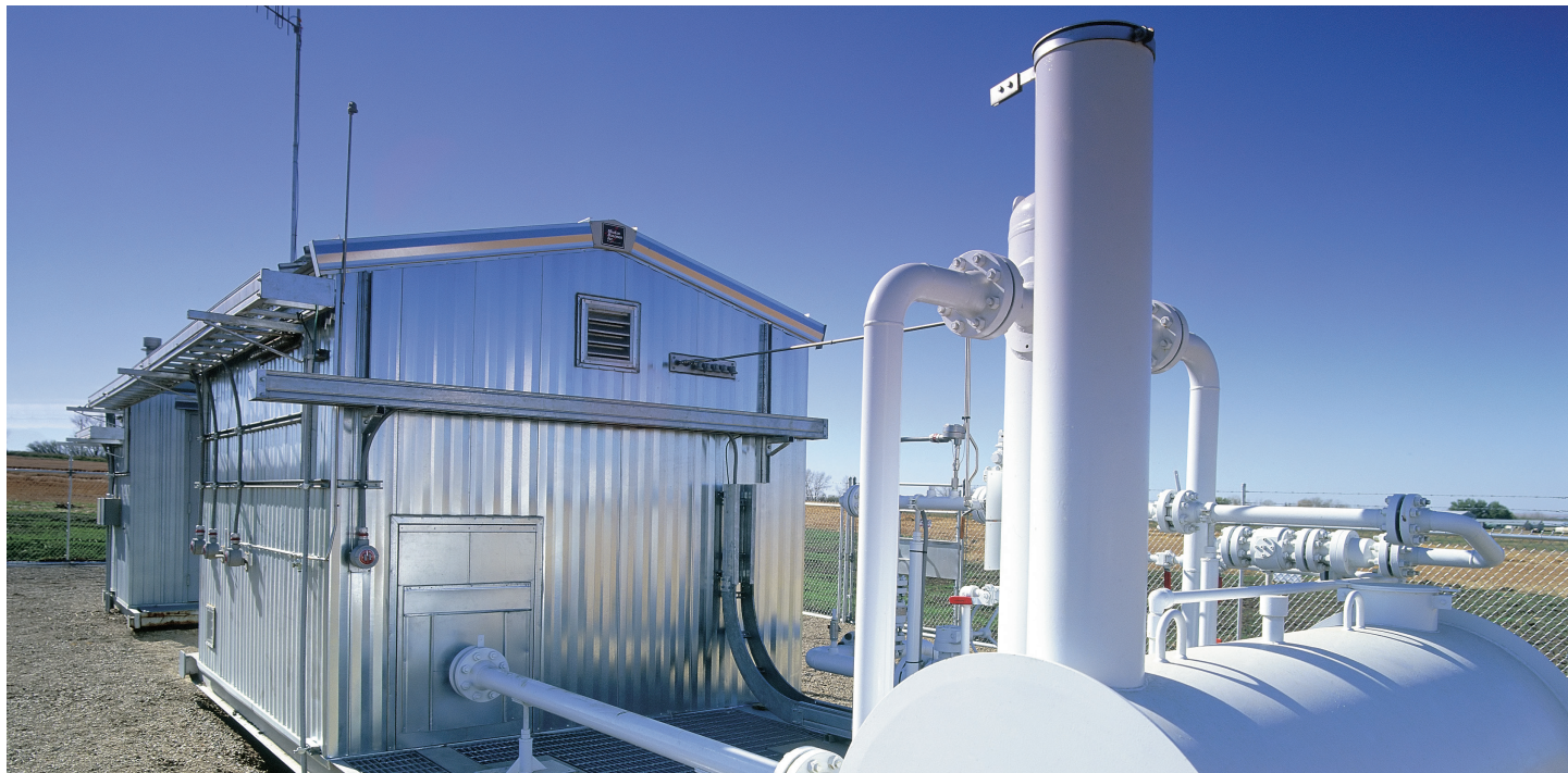
Meter stations are used to measure the volume and composition of natural gas transported through a pipeline.
