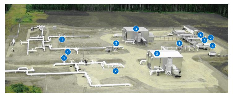
A typical compressor station includes all of the equipment illustrated here.
