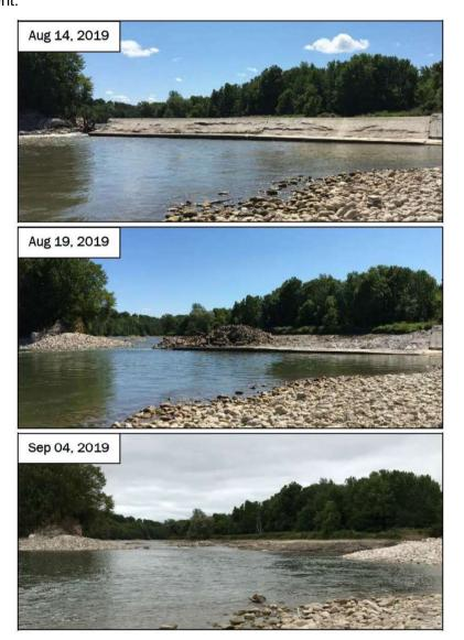
Figure 56: Truax Dam, Walkerton, ON. The original wooden dam was built in 1852 and later replaced by the concrete structure shown above in 1919. The dam posed a significant barrier to fish passage for more than a century before it was removed in the summer of 2019 over the course of 3 weeks.
