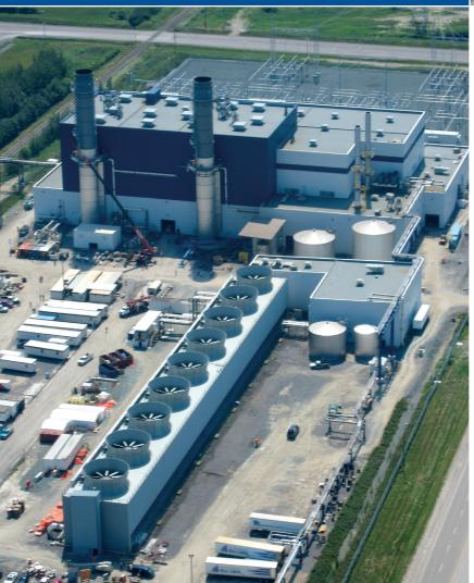
The Bécancour Power Plant is a 550 MW cogeneration facility located in Bécancour, Quebec. The facility can supply electricity to Hydro-Québec Distribution to meet electricity demands in the province of Québec and provides an important source of steam for a neighbouring company in the industrial park.
